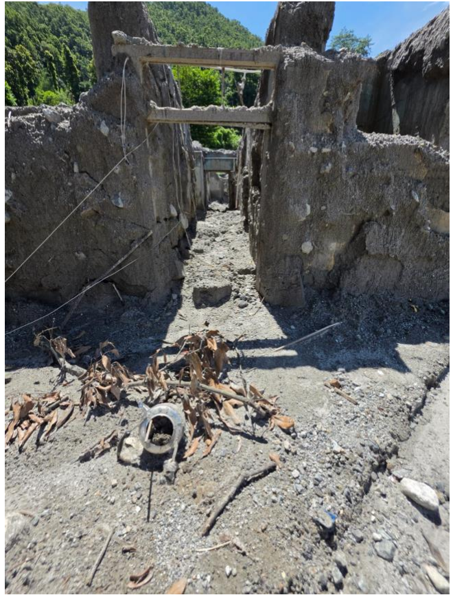
Through a doorframe that somehow survived — a corridor of rubble where rooms once were.
