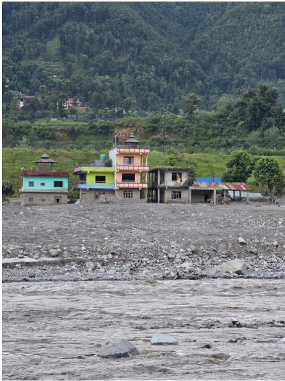
Houses along the river at Nawakot, half-buried in the silt the flood left behind.
